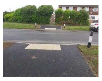
New crossing point in Old Worthing Road complete with tactile paving and dropped kerbs
