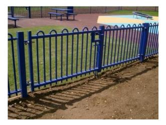
The bow top gates will be 5mtr wide and 1.45mtrs high and made from steel, with lockable slide latch and lockable drop-down bolts. All of the above information was circulated electronically to Committee for its consideration.
