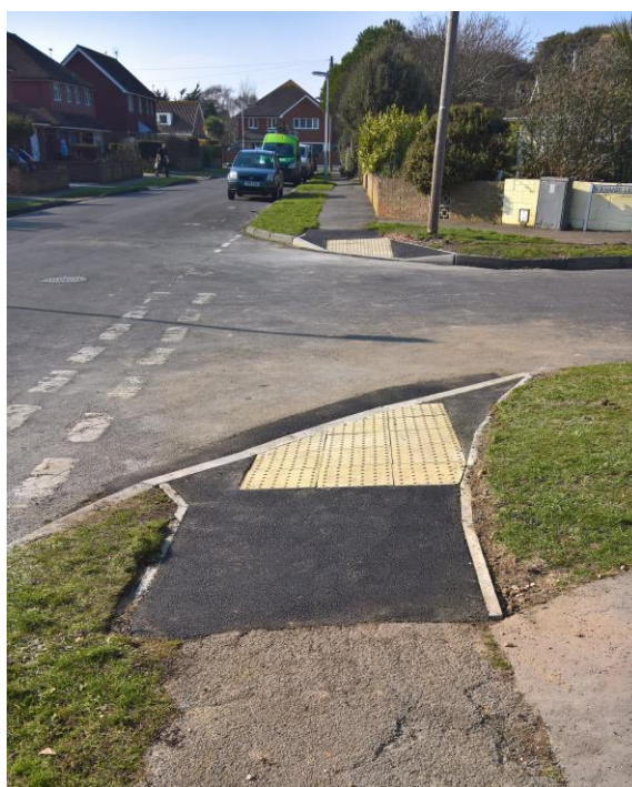
New dropped kerbs at the junction of Normandy Lane and Seaview Road.
